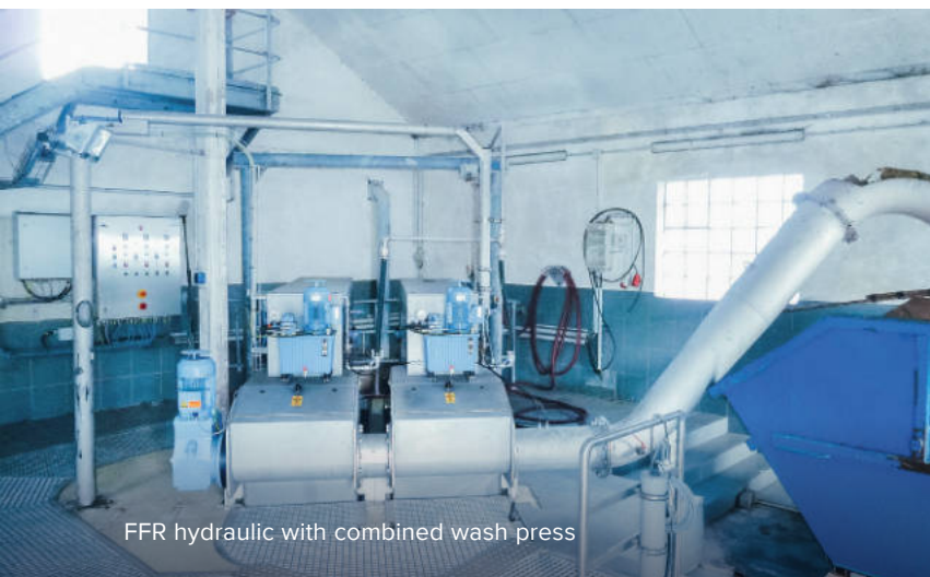
Outdoor installation in stainless steel tank
